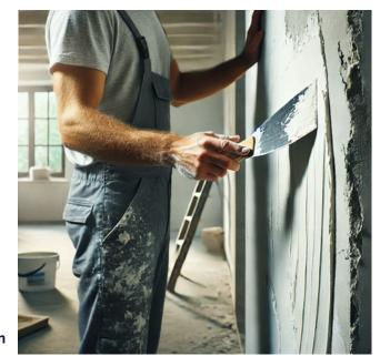
A paste of SILKCOAT-13 with Crack filling power being applied in between wall cracks
