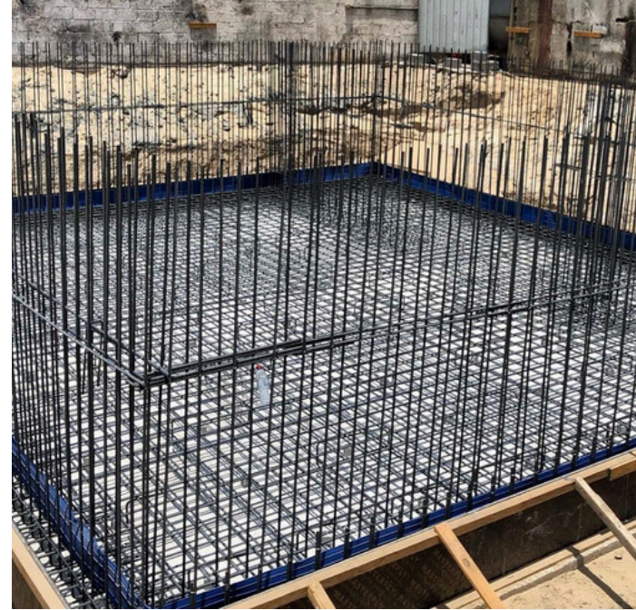
CORROSTOP-15 IN Raft Foundation
